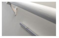
10. Secure the channel into the clips.
